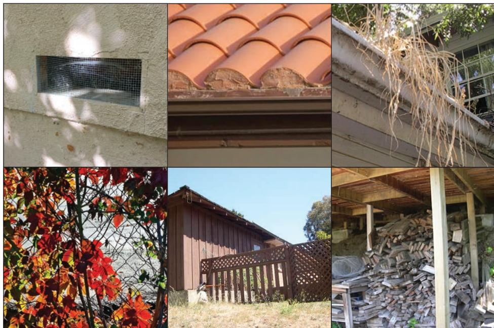
**Some tips for hardening your house against fire (clockwise from top left):** 1) Make sure all house vents have screens, roof to foundation. 2) For roofing tile, make sure ends are blocked. 3) Clean gutters of all debris. 4) Get rid of anything flammable under the deck. 5) Do not attach wood fencing to house. 6) Remove flammable plant material from wire fencing.
