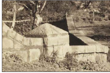
The teeth of the stegosaurus wall can be seen at top left in this portion of an image showing the stone bridge circa 1897.
