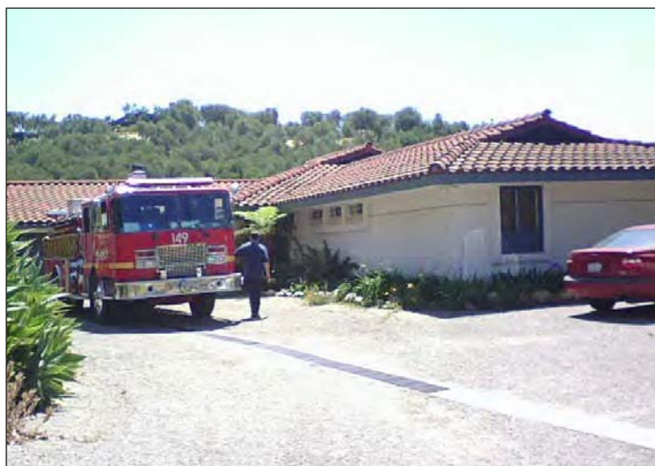
The property this home sits on got so hot that the propane tank and its safety valve parted company, but enclosed eaves, good defensible space, and a fire-resistant roof helped the house survive Jesusita, not to mention the work of firefighters on-site.
