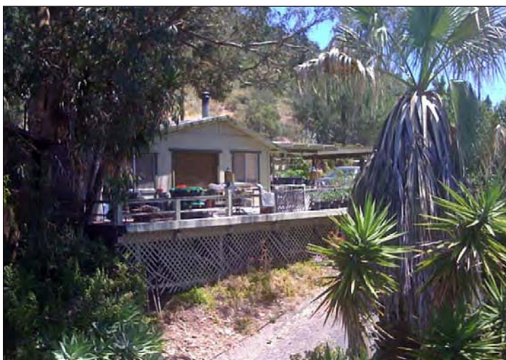
This home offered the Jesusita Fire considerable fuel in its wooden deck, nearby trees, and unfortunate location at the juncture of a couple of ridgelines. It was destroyed in the fire, and almost took the lives of two firefighters.
